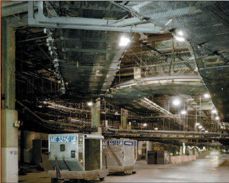
Safety netting system provided OSHA-compliant passive fall protection for personnel working above the tracks and passive overhead debris protection for personnel working below the tracks.
