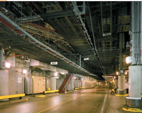
Safety netting system provided OSHA-compliant passive fall protection for personnel working above the tracks and passive overhead debris protection for personnel working below the tracks.
